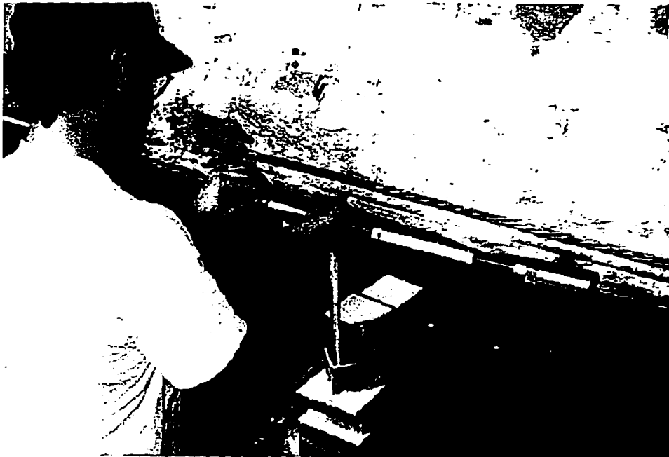
Figure 6.51 Installation of Grab-It™ Splice Assembly
