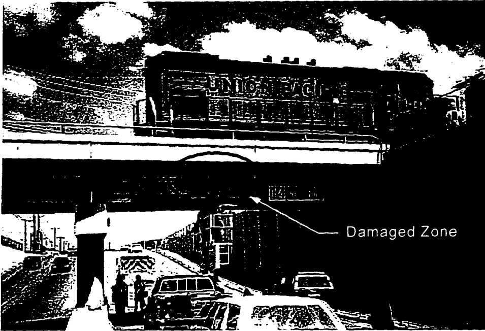
Figure 4.2 Overall View of Steck Girder In-Situ (Courtesy of the Texas Department of Transportation)
