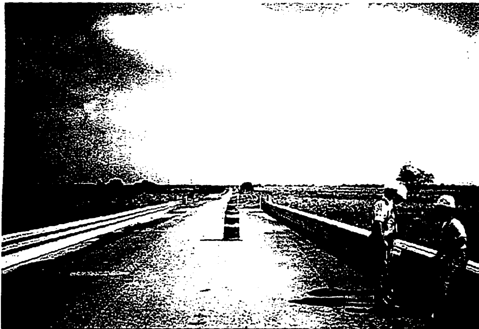
Figure 2.21 Superstructure of Waelder Bridge
